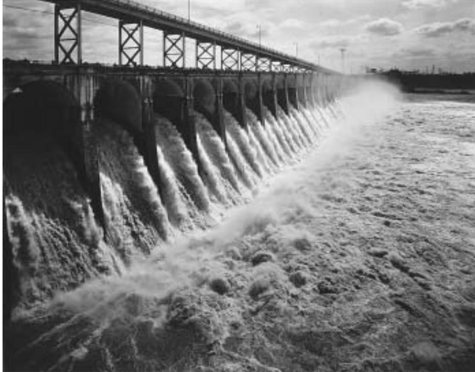
**FIGURE 11.24** The out-flow end of water-driven electric generators producing power at Wilson Dam (part of the Tennessee Valley Authority). The plant can generate electric energy at a rate of over 100,000,000 watts.
