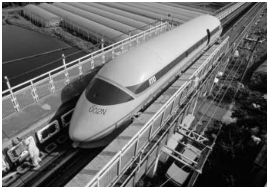
FIGURE 16.11 Japanese Mag-Lev train driven by superconducting electromagnets.
