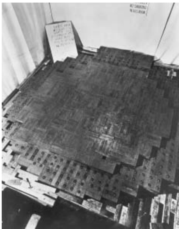
FIGURE 18.20 The Chicago pile No. 1 used by Enrico Fermi and his associates when they first achieved a self-sustaining nuclear reaction on December 2, 1942. Alternate layers of graphite, containing uranium metal and/or uranium oxide, were separated by layers of pure solid graphite blocks. Graphite was used as a moderator to slow down neutrons in order to increase the likelihood of fission. Courtesy of Argonne National Laboratory.
