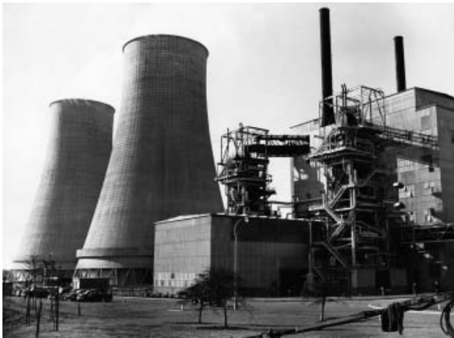
FIGURE 18.23 Reactor Number One at Great Britain's first nuclear power station at Calder Hall (opened in 1956). The large towers are cooling towers. The reactor is in the large building.
